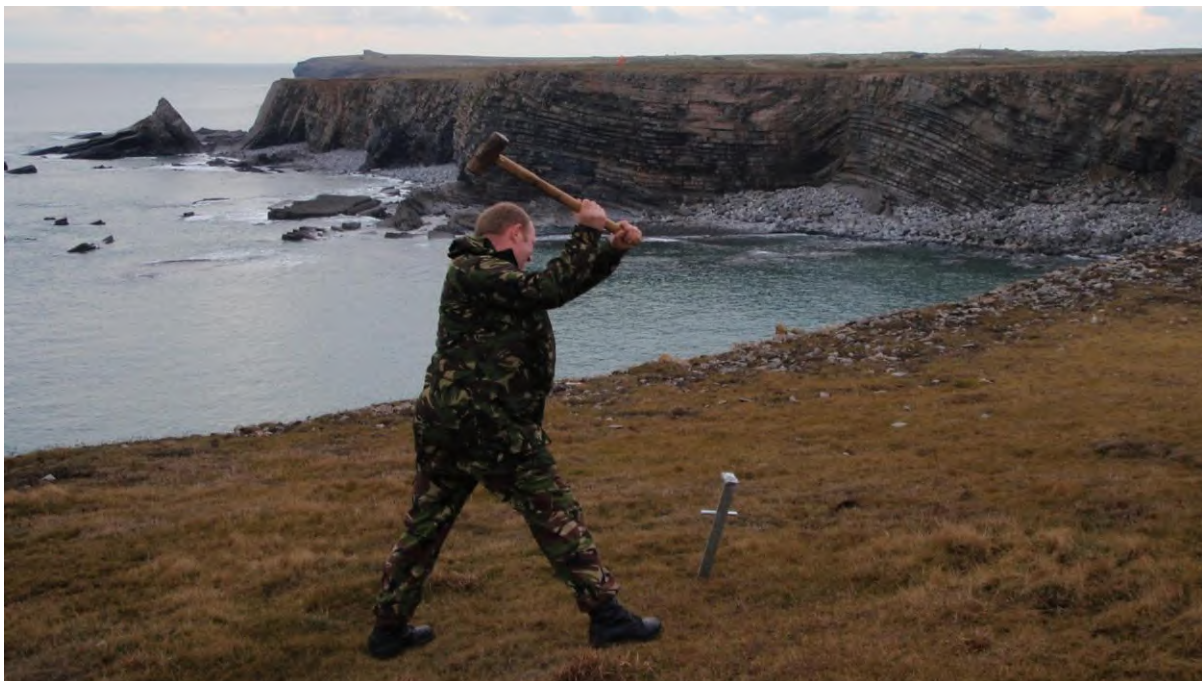
Placing new BMC belay stakes at Range West (photo: Steve Quinton)
